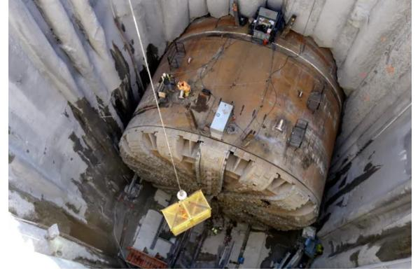
A worker inside a metal cage is lowered into an access pit holding the damaged digging machine for the Highway 99 tunnel project Monday, March 9, 2015, in Seattle. The single-bore technology, seen here during a Seattle highway project in 2015, has never been used to mine a subway tunnel in the United States. (AP Photo/Elaine Thompson)
